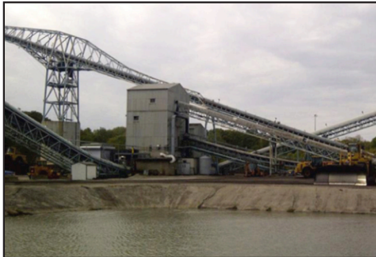
Maintaining proper lubrication for conveyor bearings was difficult.
